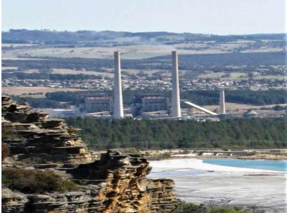
*Photo: Wallerawang Power Station when operating showing the 176 metres high Unit 7 & 8 stacks, and smaller 80 metre high stack of the old Wallerawang Plant A on the right. Note Wallerawang township in the background, and smoke emissions blowing at almost right angles from stacks at 1016m elevation.*
